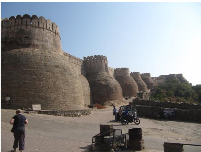
Part of the wall
