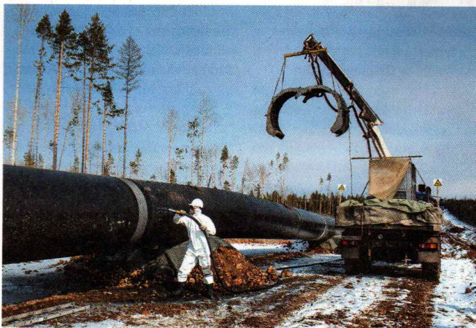
A worker repairs an oil pipeline owned by Russian firm Gazprom
